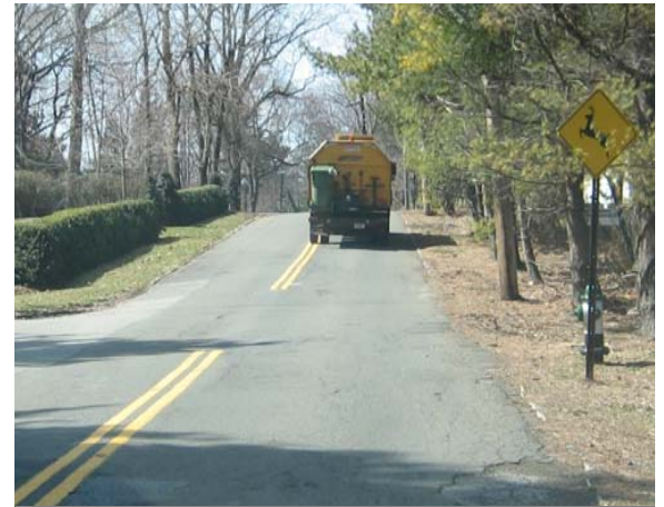
Proposed new Sidewalk on West Ardsley Av Street width: 20'-4" Verge width 4' Cars: 115 vph Pedestrians: 0 qualifying pph + 57 older pph
